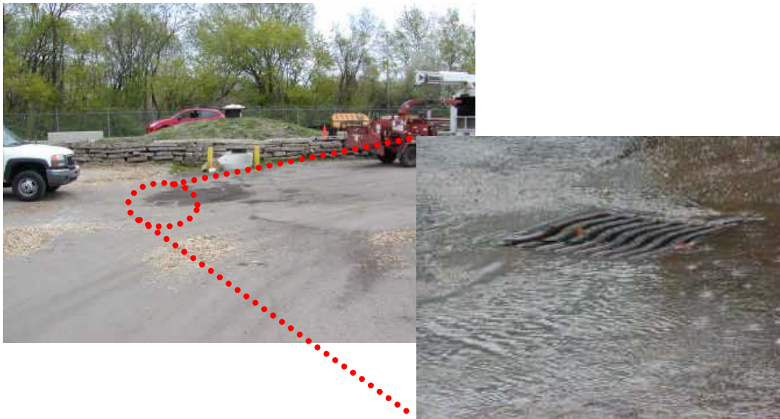
(a) City of Kalamazoo Public Services Building at 415 Stockbridge Avenue
