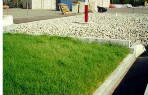
(b) Altadena Maintenance Station
