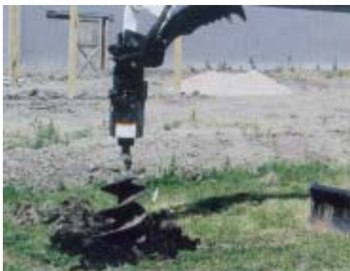
Fig. 46 View of auger
