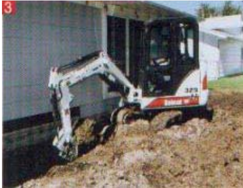
Fig. 42 View of small-sized back hoe
